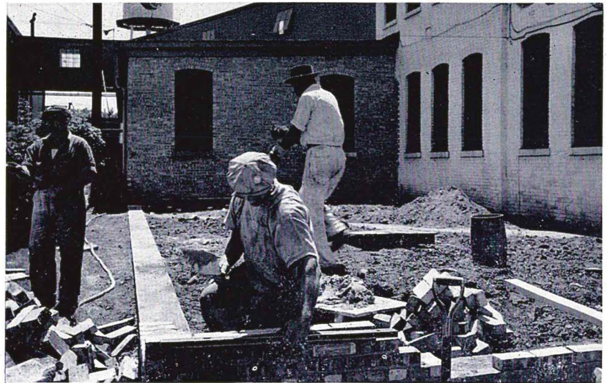
Laying the first bricks for the new office addition structure. The building will be two stories high at the side shown in the illustration with a second story addition extending over parts of the tool room and machine shop at the south end of the present off. ce.
